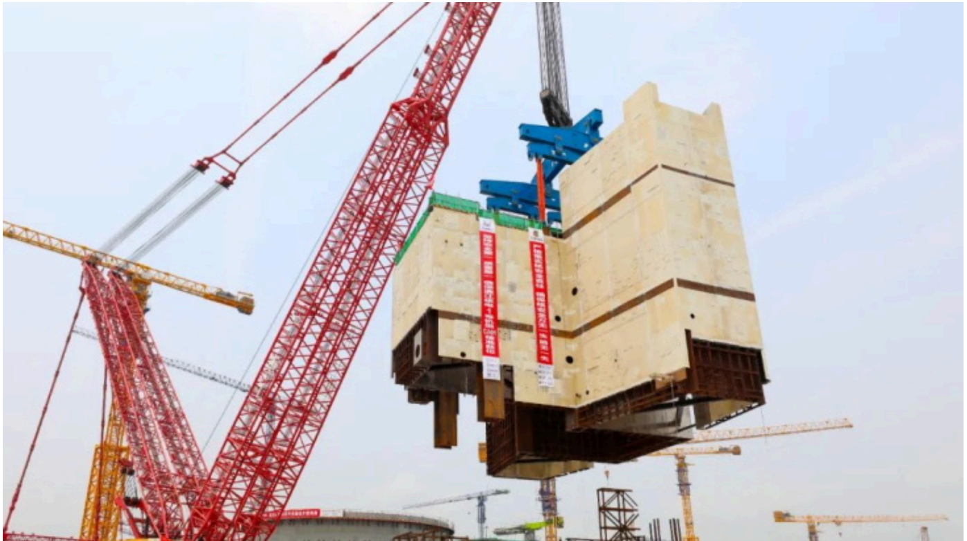
The CA01 module is hoisted into place (Image: SNERDI)
